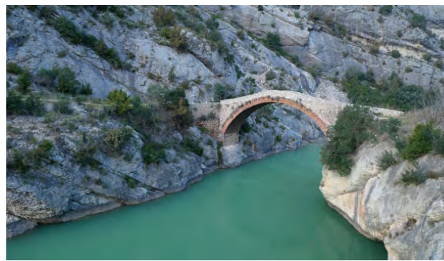
The Noguera Pallaresa river on its way through the old Terradets bridge.
